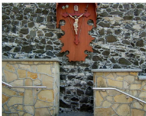
Fig. 13. The wall near the main stairs leading to Basilica (point 7)
